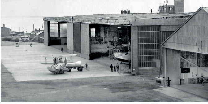
Naval Air Station, Caquot shed, 1936
